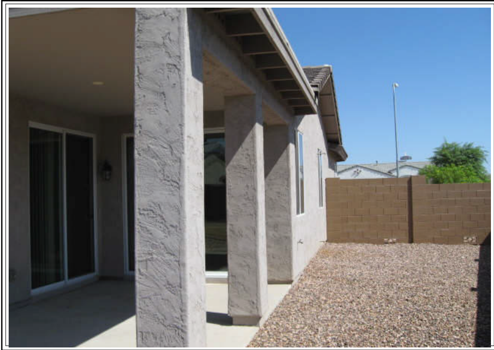
EAST SIDE OF SUBJECT
